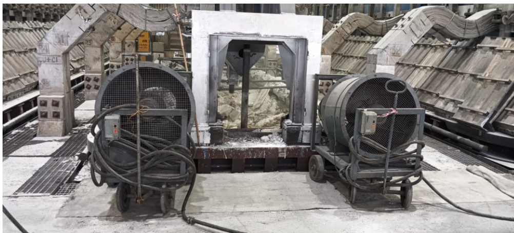
Figure 1. Air cooling by high-capacity fans in 235 kA potline.
