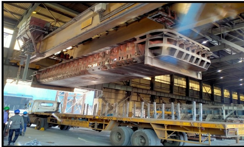
Figure 4. First ever pot shell removal for off-site maintenance.
