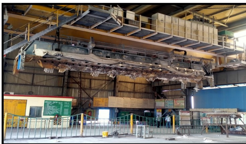
Figure 3. First ever PSS removal for off-site maintenance.
